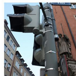
Fixation of traffic signal device
