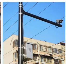
Fixing of surveillance camera
